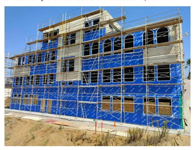
Stucco work continues, particularly on the South elevation where much of the wood rot has been repaired and replaced.
